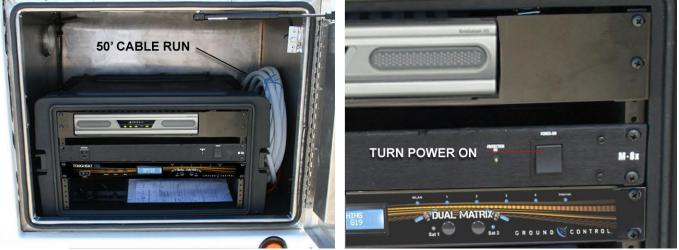
**STEP 10 – TURN ON ELECTRONICS**. Inside of the electronics case is a portable 6RU rackmount case with an 50 foot cable run that allows you to move the electronics a distance from the trailer. The electronics case includes the iDirect satellite gateway, the 8 AC plug power conditioner, and the Toughsat wireless controller. Both the gateway and controller should power on (lights will appear) with the single toggle switch on the power conditioner.
