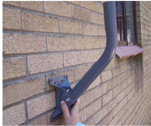
Figure 4-3 – Pole Assembly
